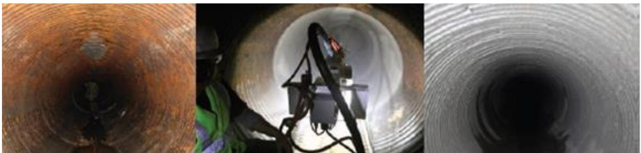
Figure 2: From left to right (a) Leaking storm water culvert (b) Centrifugal application of GeoSpray™ (c) Completed Repair<sup>11</sup>
