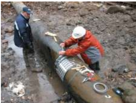
Installing the RidgeBack™ system
