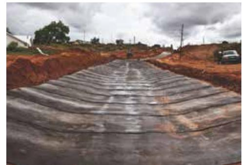
The entire 12,000 square feet of Concrete Cloth material was installed in one day, despite rainy conditions.
