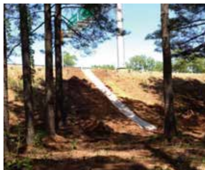
Concrete Cloth material installed pre-landscaping
