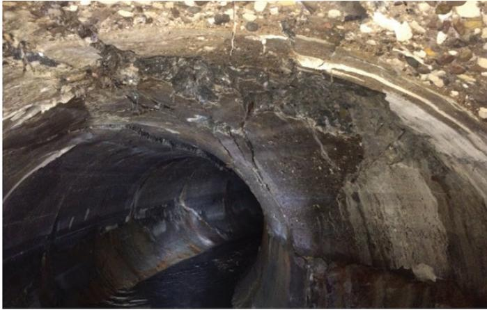
Damaged and corroded sewer interceptor under Tireman Avenue.
