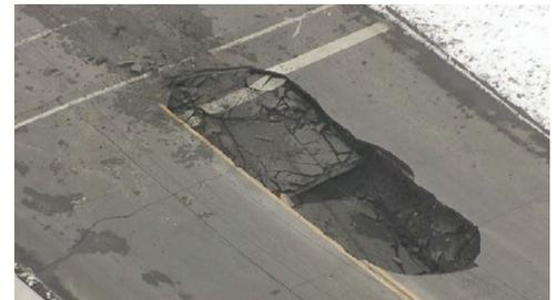
Sinkhole on Tireman Avenue caused by damaged interceptor.
