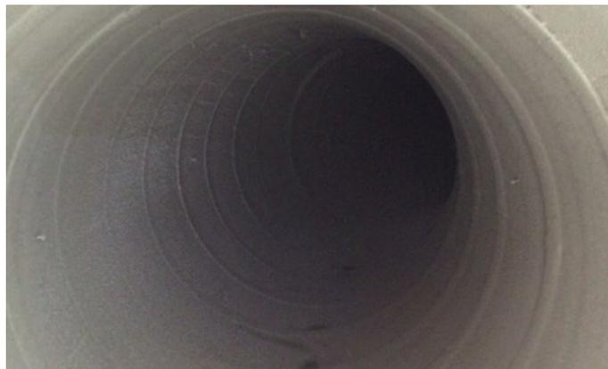
Completed rehab of curved section of interceptor.
