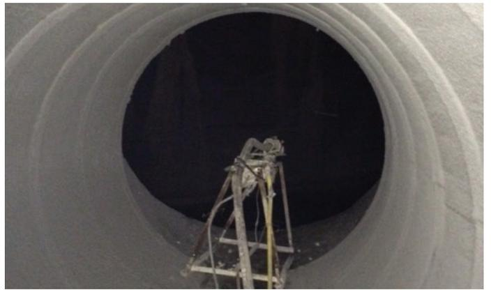
GeoSpray coating for strength and corrosion resistance over steel.
