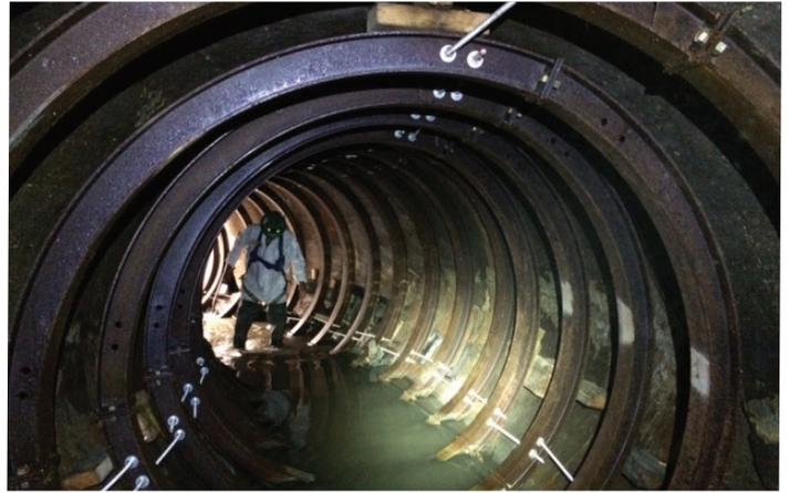
Lattice girders installed to shore up collapsed structure.
