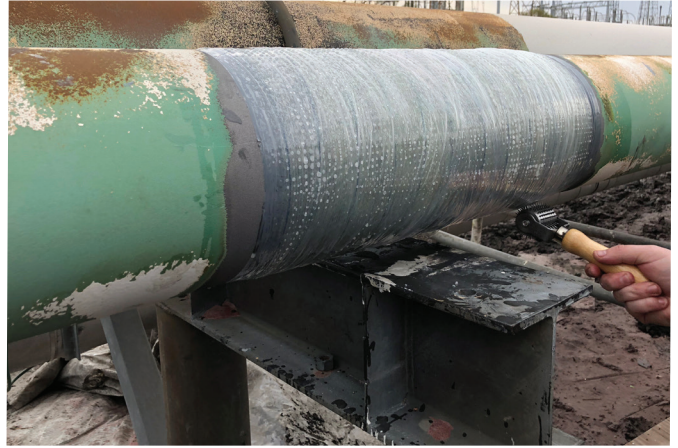
FormaShield installation in progress with perforating constrictor wrap.
