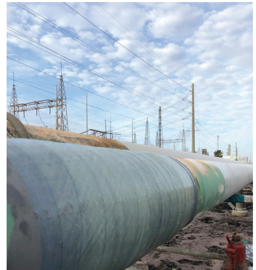
Completed FormaShield repair.
