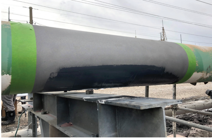
EP-420 filler material applied.
