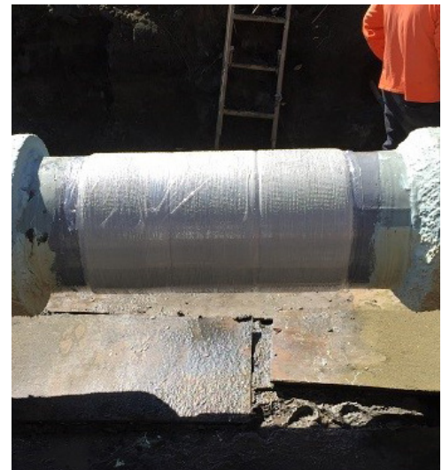
Completed A+ Wrap installation
