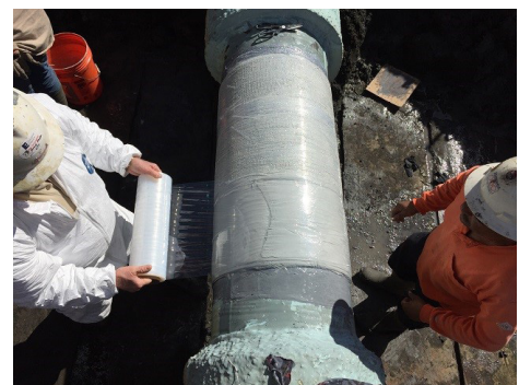
A+ Wrap installation with Constrictor Wrap
