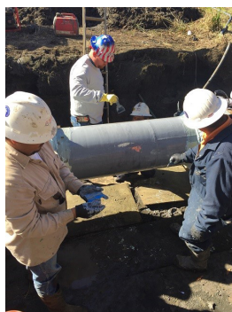
Application of PPR epoxy
