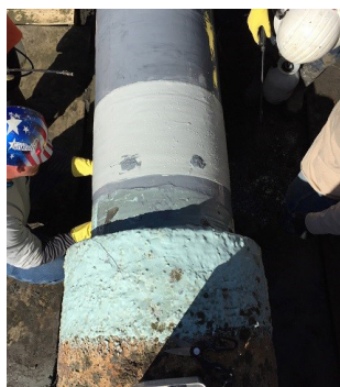
Installing ILI markers
