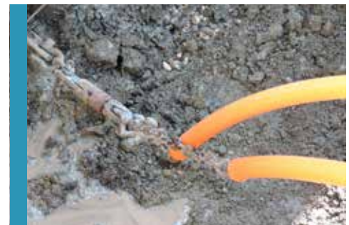
VIS DIVIDE BEING PLACED
