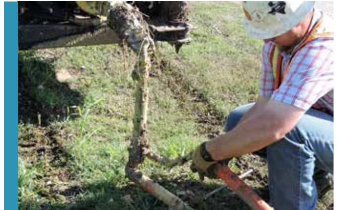
VIS DIVIDE - 2 CONDUITS PLACED SIMULTANEOUSLY
