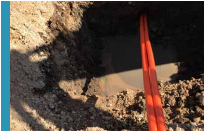
VIS DIVIDE READY TO BE PLACED
