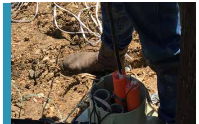
CABLE PLACED IN VIS DIVIDE
