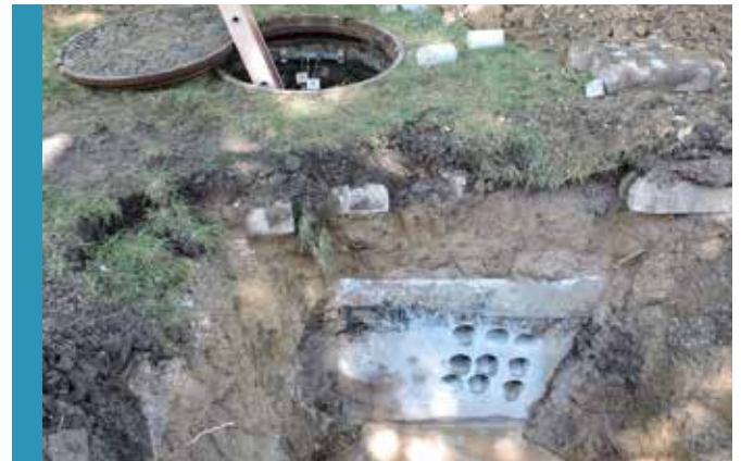
HOLES DRILLED FOR MAINTENANCE HOLE ENTRY
