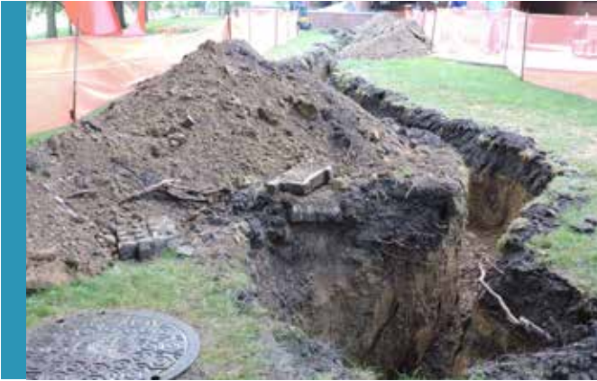
TRENCH READY FOR INSTALLATION
