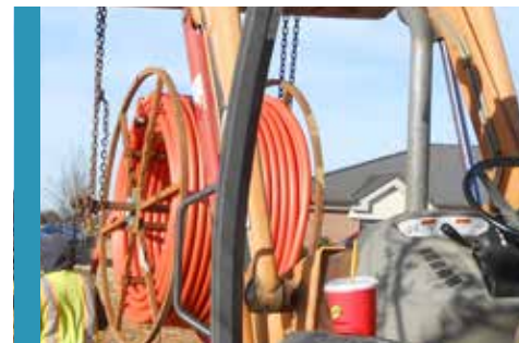
VIS DIVIDE READY FOR INSTALLATION
