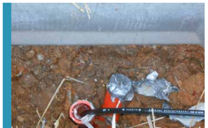
CABLE PLACED IN VIS DIVIDE
