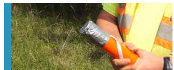
Secure Pull Tape to Conduit
