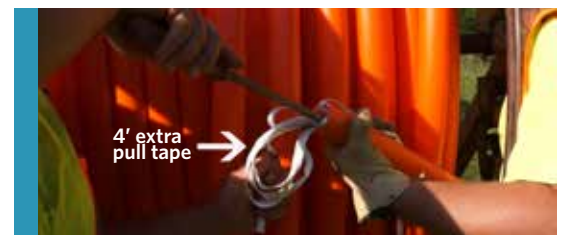
Push Excess Pull Tape into Cells
