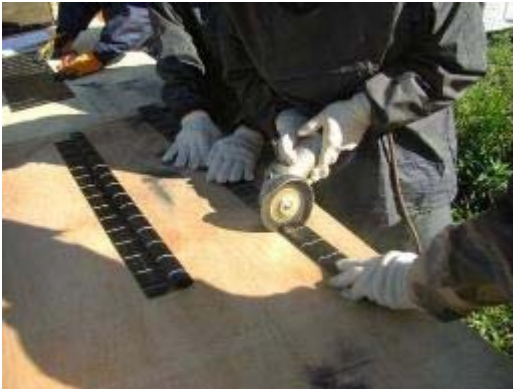
Cutting Strand Sheets with grinder
