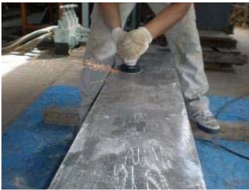
Using a disk grinder to prepare the surface of the steel
