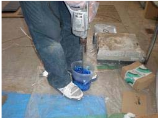
Mixing RenewWrap Strand Sheet Adhesive (FB-E7S)
