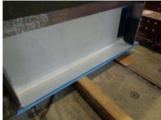
Completed fillet ready for fabric reinforcement
