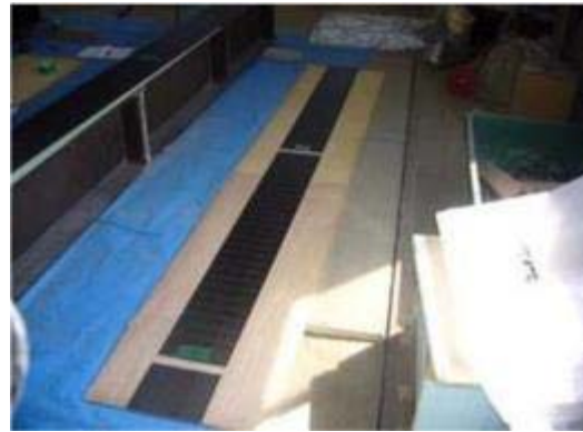
Cut strand sheets stacked ready for installation
