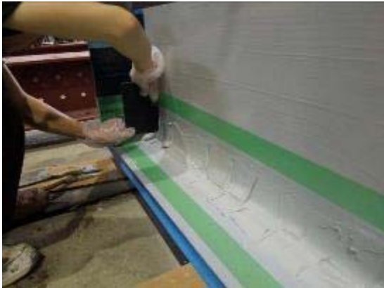
Creating a fillet with the filler putty
