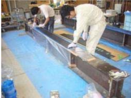
Placing Strand Sheet onto surface
