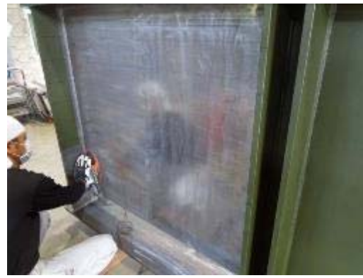
Cleaning surface with acetone
