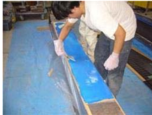
Applying Adhesive to primed steel surface
