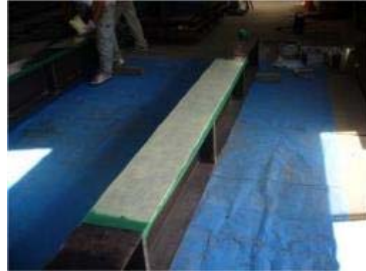
Primed surface curing before application of Strand Sheets
